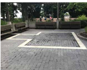
Typical perimeter concrete installation
